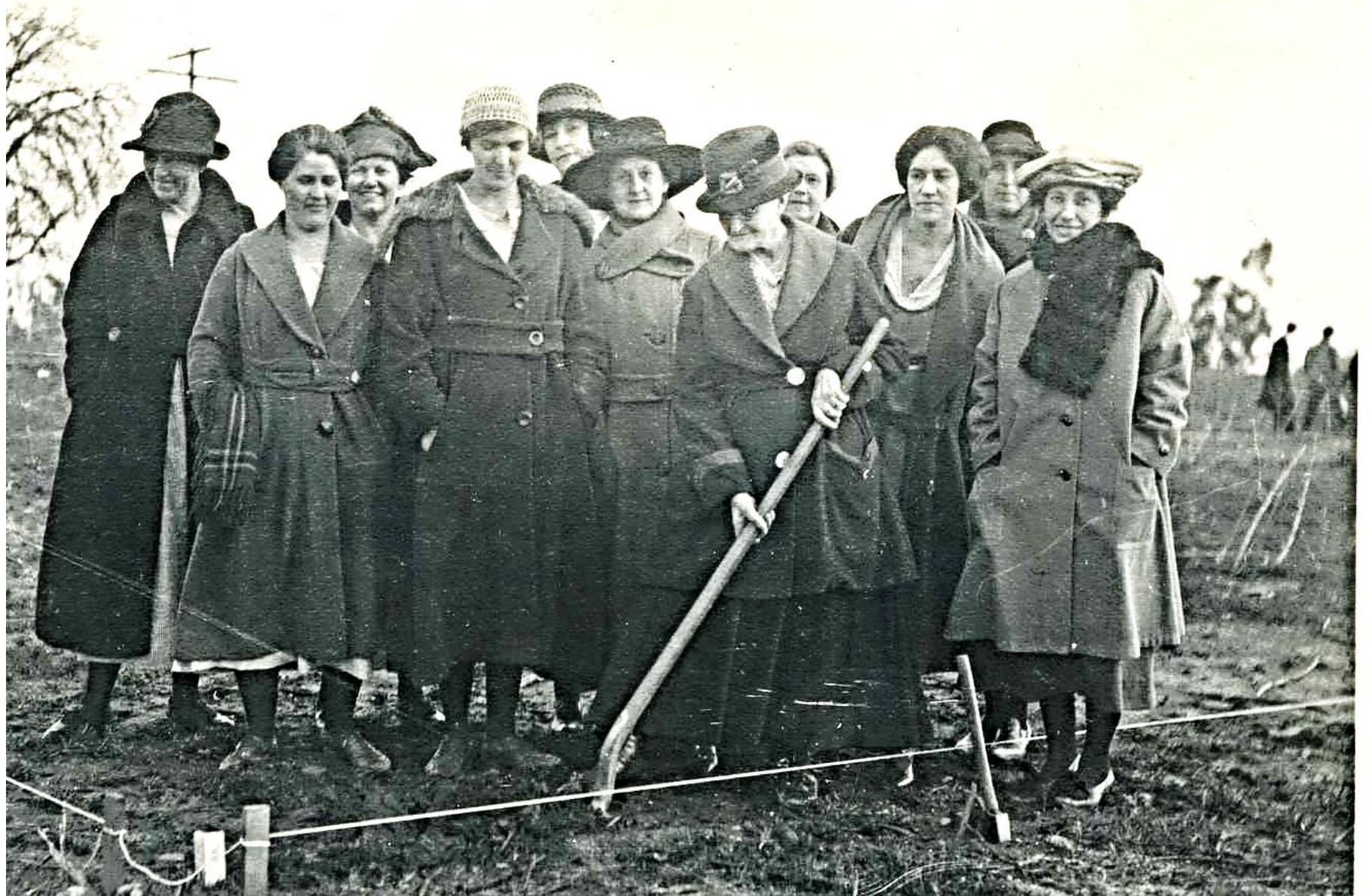
Breaking Ground for the Club Building
